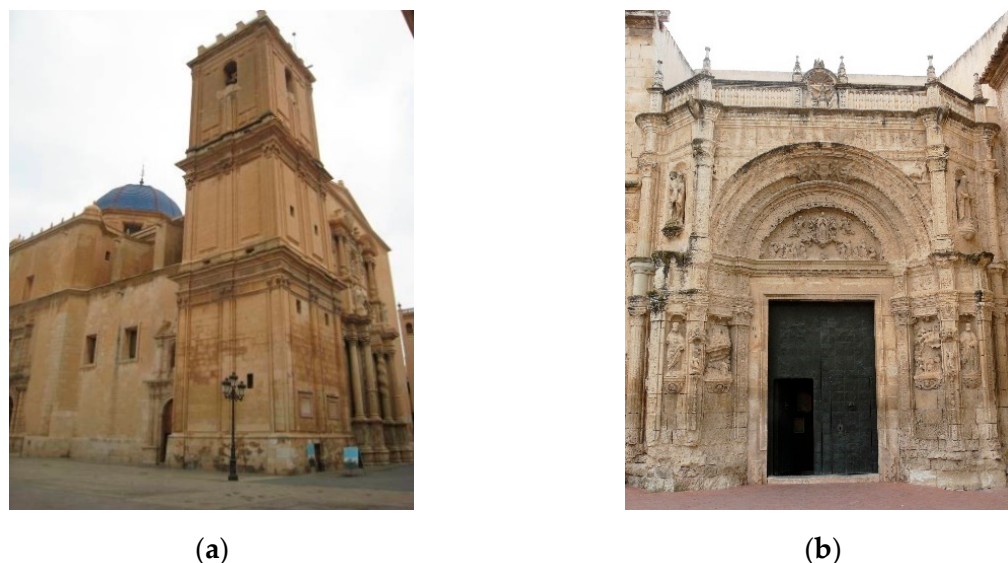
Figure 1. Historical buildings built with calcarenite stone; (a) Basilica Santa Maria (SM) in Elche (Serravallian stone); (b) Church of Nuestra Señora de La Asunción in Biar (IB) (Eocene stone).
