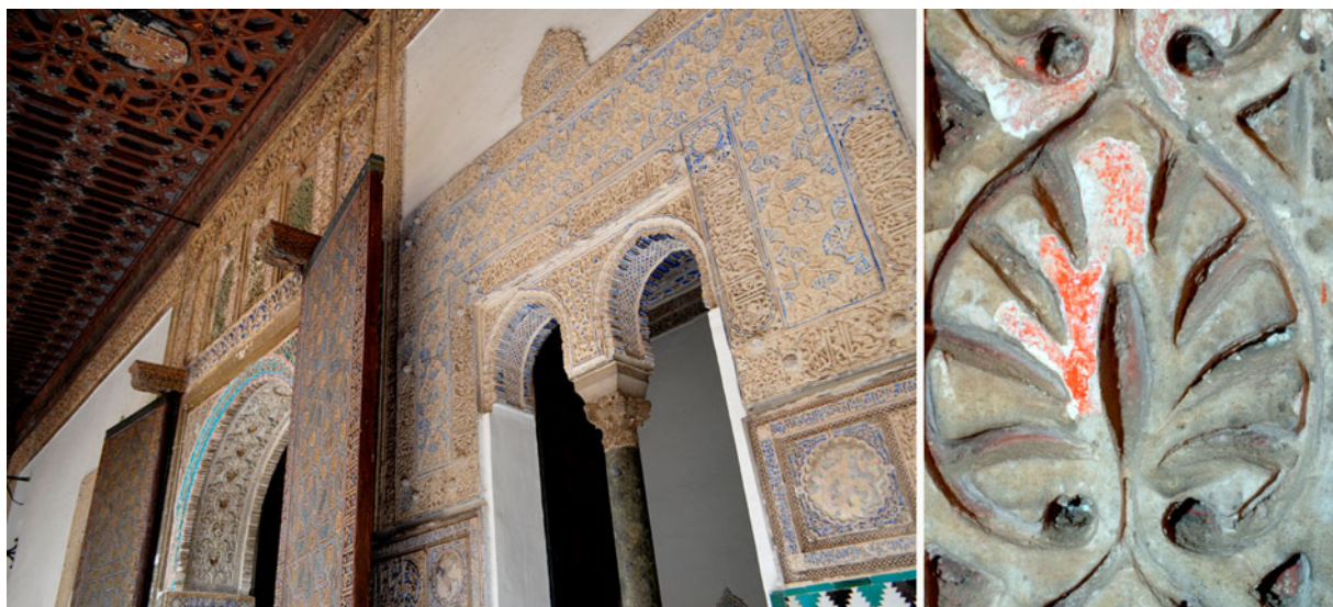
Figure 1. Left: Plasterwork on the south-eastern wall of the Courtyard of the Maidens, where the original blue polychrome persists. Right: Detail of results of a cleaning test on one area of this plasterwork, which decorates the main entrance to the Salón del Techo de Carlos V , where some remains of the original red polychrome can be seen.
