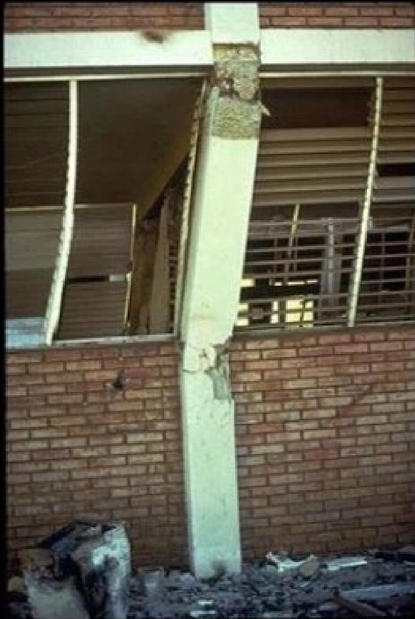
short column damage
