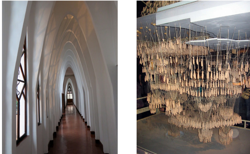
Fig. 1. Left: Corridor in the Colegio Teresiano, Barcelona [41]. Right: a hanging model of the church of Colonia Güell used by Gaudí with funicular structures [42].
