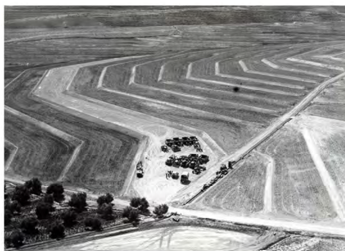
Figure 7. Extensive efforts to move earth with tractors for the adaptation of the topography to implement the new agricultural division of land in terraces (ca. 1955–1960). Source: Archive of the Spanish Ministry of Agriculture; File: 19333-c8-cd6.
