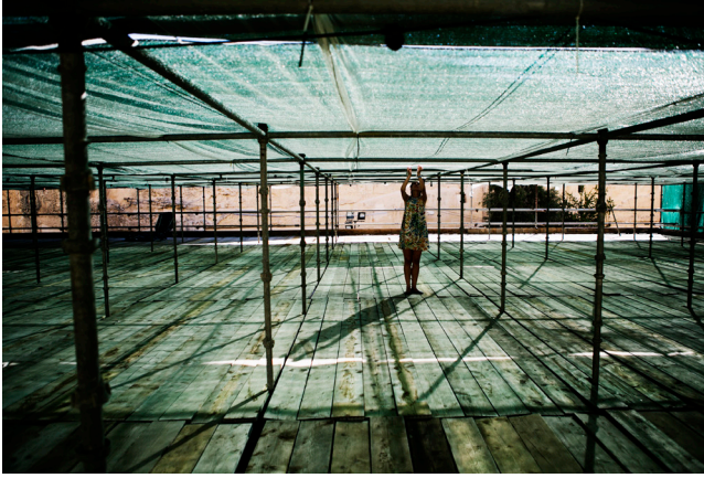
Figura 29. Montando el accommodation. EASA Malta 2015 13
