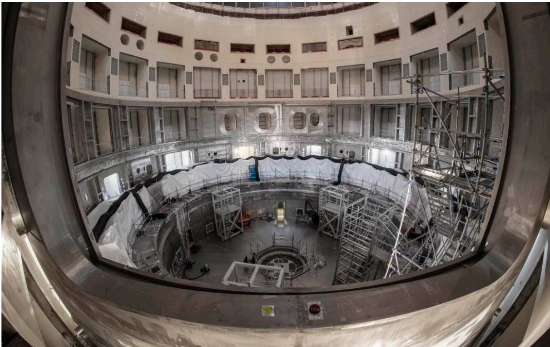
Figure 2. ITER under construction. Credit © ITER Organization, http://www.iter.org/ .
