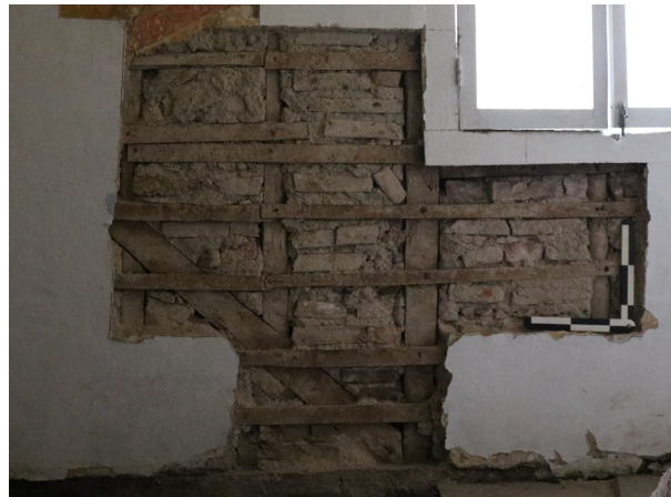
Figure 2: Coimbra's "medieval house" (survey 1) Source: A. Ginja (2017)
