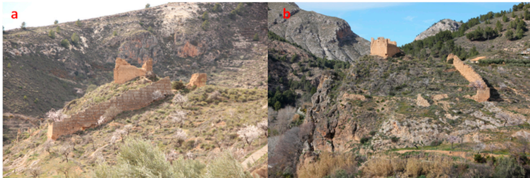
Figure 4. View of the remains of Lojuela Castle from its (a) eastern and (b) southern sides. Source: PREFORTI project.
