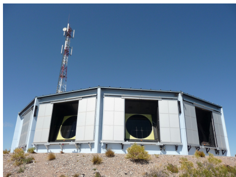
Figure 2.5: FD building at Los Leones during the day. Shutters are open because of maintenance. Behind the building there is a communication tower.
