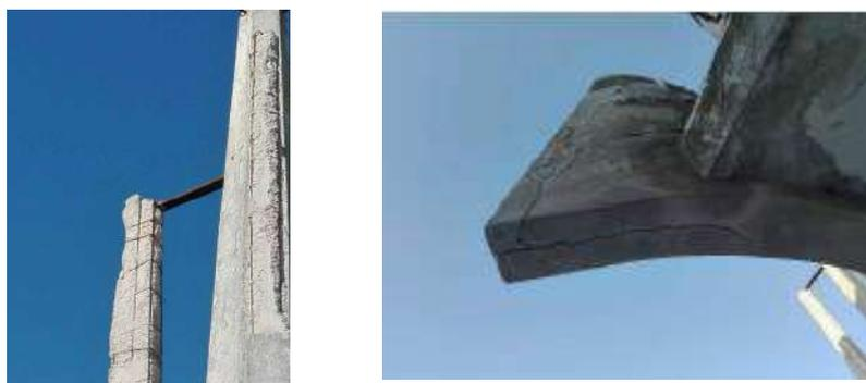
**Figure 3.** Detail of damages observed on the r.c. structures on the Church of Santa Maria Assunta bell tower.
