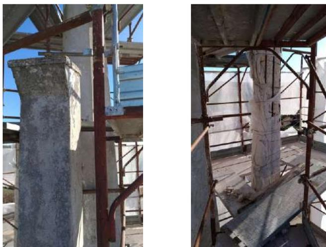
Figure 4. Details of coatings and scaffoldings before the retrofitting intervention.
