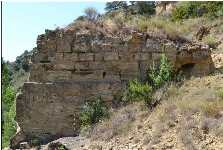
Fig. 3. Western abutment of a medieval bridge in Lizana (Barbuñales, Huesca)
