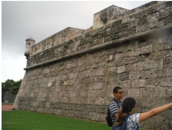
Figura 106. Baluarte Santa Catalina Garita
