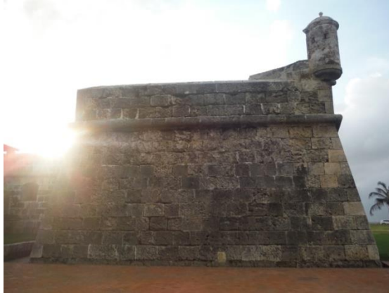
Figura 105. Baluarte Santa Catalina Garita
