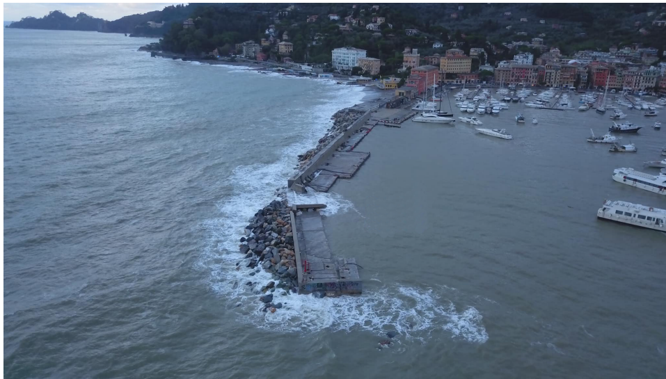
FIGURE 1: Scheme of the collapse of the main armor layer of a rubble mound breakwater.
