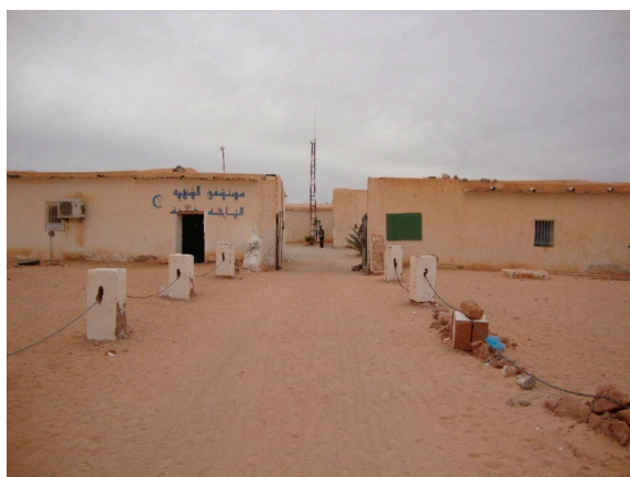
Figure 4. Regional hospital at the wilaya Awsard. Source: author's own photo.
