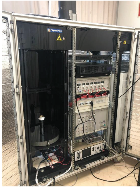
Figure 3.2. Raman lidar MULHACEN system working at IISTA-CEAMA facilities in Granada (Spain).
