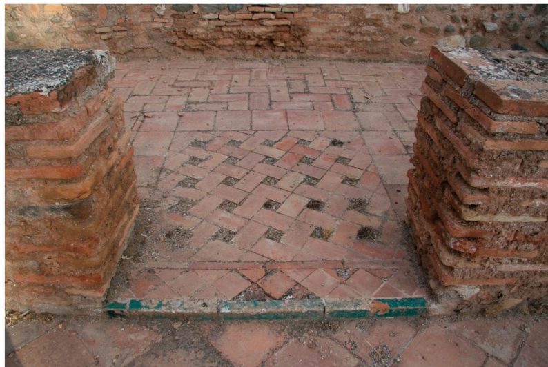
Figure 6. Reconstructed almatraya from the Nasrid period with missing glazed ceramic pieces from one of the houses alongside the Gate of the Seven Floors (Puerta de los Siete Suelos). © María Elena Díez Jorge, 2017.
