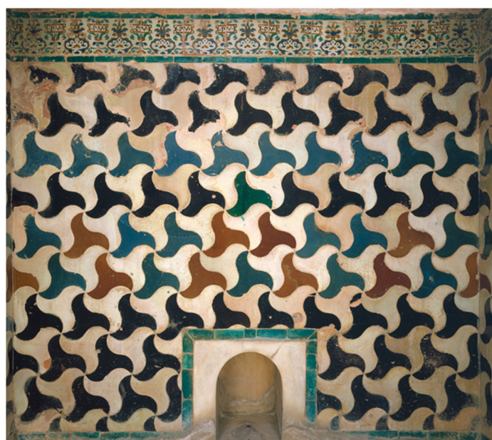
Figure 12. Detail of alicatados in the Comares Baths, built in the 14th century, although featuring some ceramic pieces from the 16th century which are clearly visible in the arista tiles from this period bearing the initials of Plus Ultra. © María Elena Díez Jorge, 2014.
