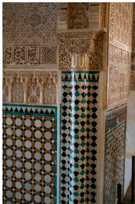
Figure 8. Columns faced with alicatado pieces, cut in a curve. Comares Palace, 14th century. © María Elena Díez Jorge, 2018.
