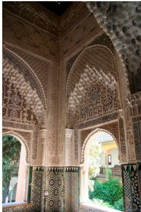
Figure 2. Arab sources from the Nasrid period already highlighted the quality of work of the master craftsmen in the alicatados and plasterwork. Plasterwork and alicatados in the Lindaraja balcony, Palace of the Lions. © María Elena Díez Jorge, 2014.
