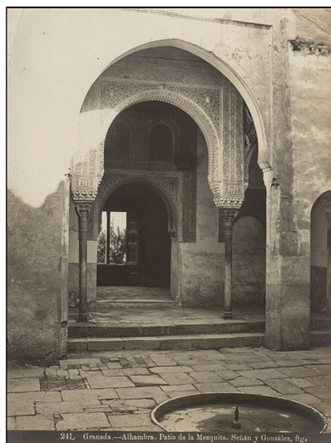
Figure 22. Portico and Cuarto Dorado before dismantling the 16th century arches. The photograph shows the alicatado work below the mullioned window, looking toward the east. Photograph by Rafael Señán y González (undated). © Archivo del Patronato de la Alhambra y Generalife, Photograph Collection, F-038828.
