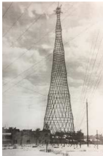
Figure 14. Six-section Tower. Shabolovskaya str. Radio tower of Komintern in Moscow. General view. Engineer V.G. Shukhov, 1922
