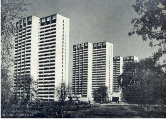
Figure 166. Residential building, type I-700A. 1980-1990.
