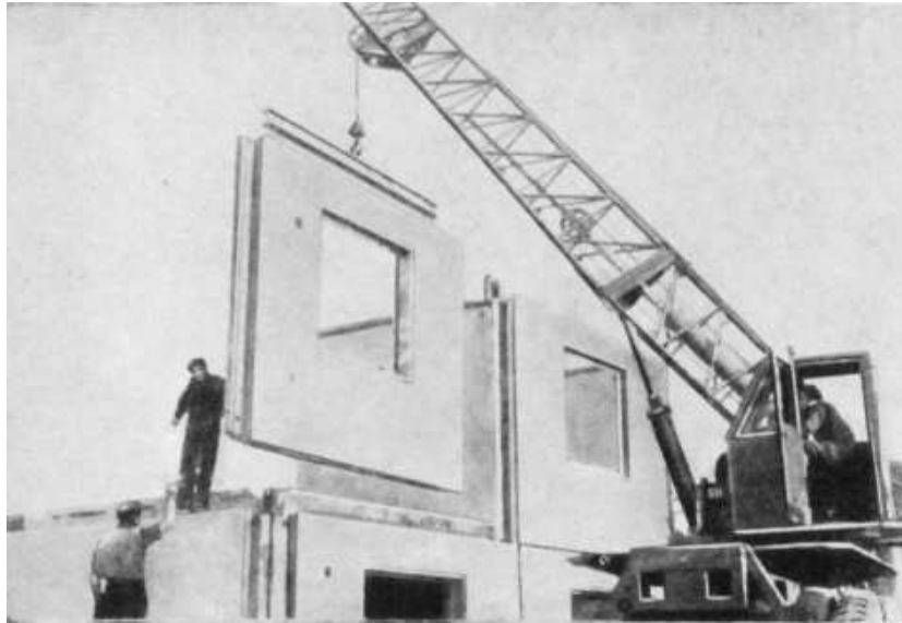
Figure 129. Pre-fabricated panel system construction.
