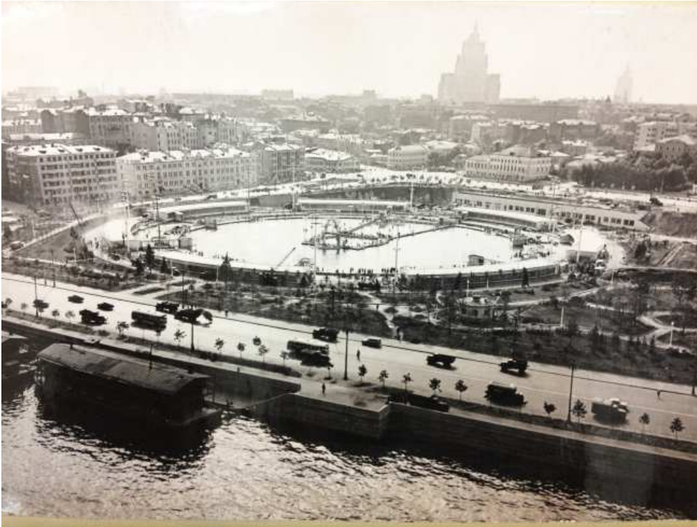
Figure 125. Swimming pool, on Kropotkinskaya Quay, which recycled the foundations of the Palace of the Soviets. General view. Arc. D. Chichulin, V. Lukyanov, N. Molokov, eng. N. Vishnevskiy. 1960
