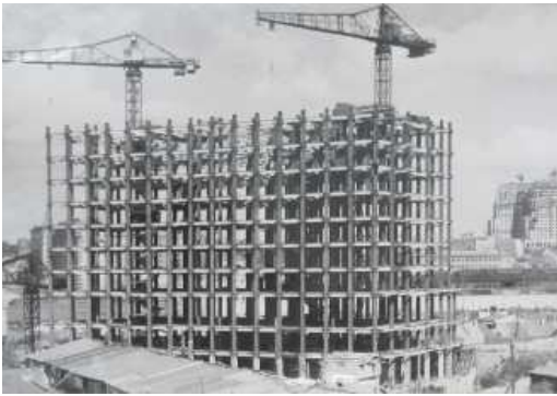
Figure 128. Hotel on Dorogomilovskaya quay. Framework construction process. Arc. A.G. Mordvinov. 1951
