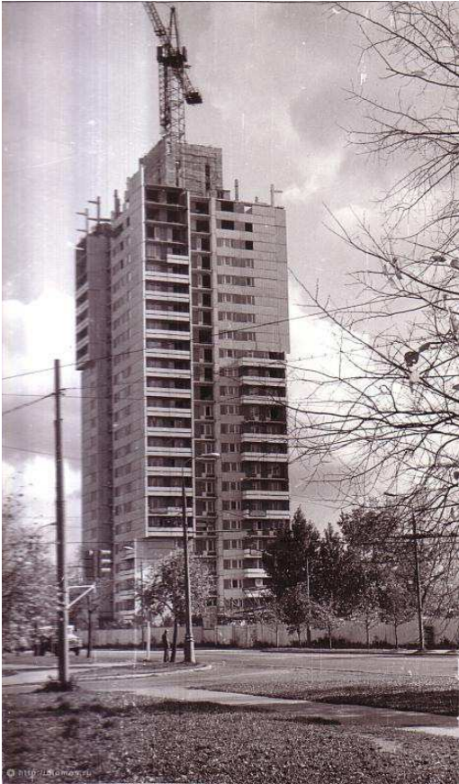
Figure 161. I-521A type of residential building. Marshal Jukov Avenue (photo from 1978)
