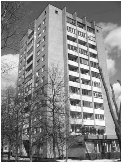
Figure 152. Brick tower on Gamalei street, h.23K2. 1975
