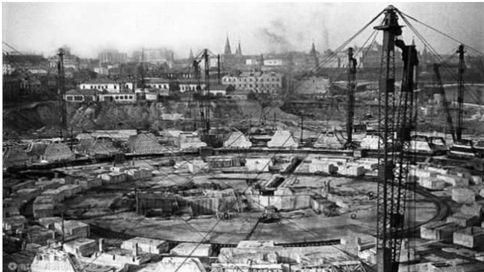
Figure 63. Construction of the Palace of the Soviets foundations.
