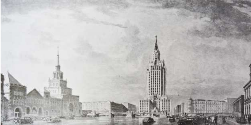
Figure 111. The building of Leningradskaya hotel on Komsomolskaya square. Arc. L.M. Polyakov, A.B. Boretskiy. 1956
