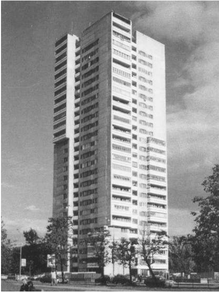
Figure 163. Leninskiy Avenue 121/1. 1967. I-521-A building type
