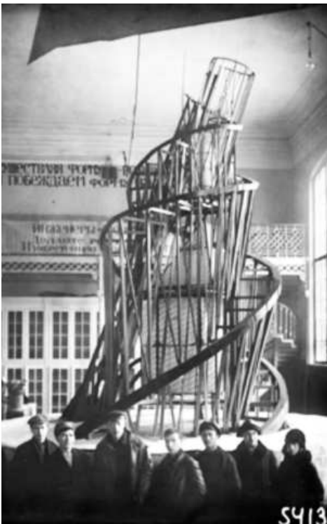
Figure 8. V. Tatlin, The model of the Monument to the Third International in the Study of Materials, Volume & Construction, in the Mosaics studio in the former Academy of Arts, Petrograd, November 1920.
