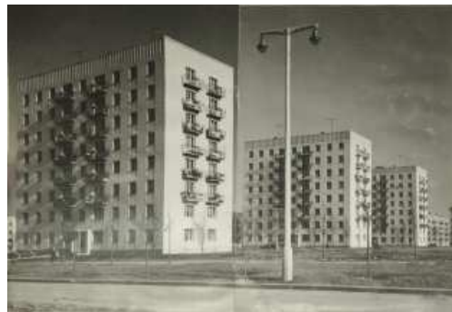
Figure 149. The project team led by the architect N. Osterman. An experimental quarter number 9. Novye Cheremushki, Perspectiv view. 1958
