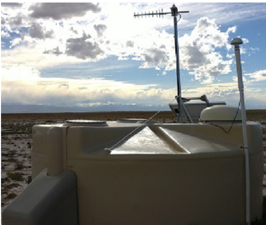
(c) EASIER antenna mounted on a surface detector.
