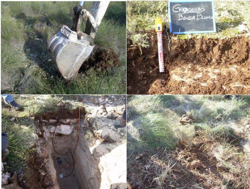
Figure 8. Instalation of vertical Co2 profile in January of 2010
