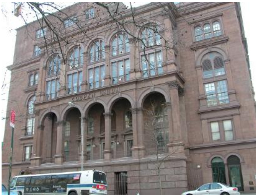
Figure 2-2. Cooper Union for the Advancement of Science and Art Foundation Building (1858) after restoration
