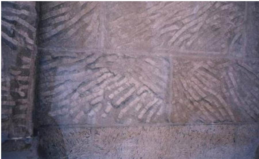
Figure 2-3 Portland Brownstone jack-hammered surface of the Cooper Union for the Advancement of Science and Art Foundation Building (picture provided by Ivan Myer)
