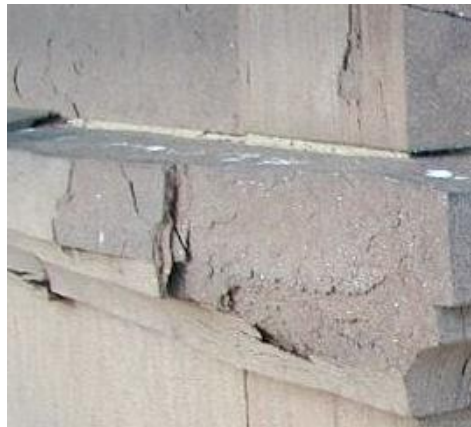
Figure 5-1. Possible case of buckling due to clay swelling. Surface of Portland Brownstone front in the Victoria Mansion, Portland (Maine). The picture was kindly provided by I. Myjer.
