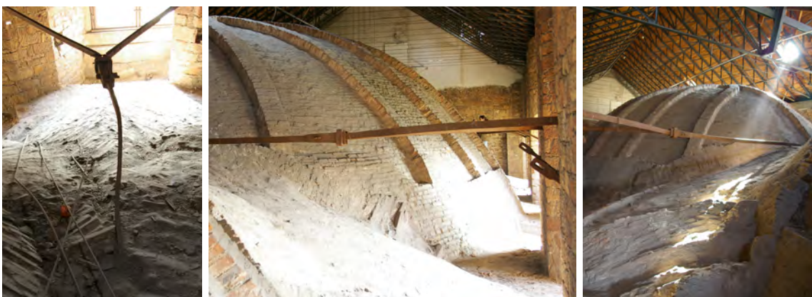
Fig.2. The extrados of the construction of the Chapel of the Residenz in Würzburg.
