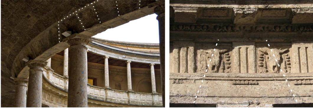
Fig. 86 and 87. Joints of the stone and contradiction of the decorated metopes and triglyphs relationship with the constructive joints.
