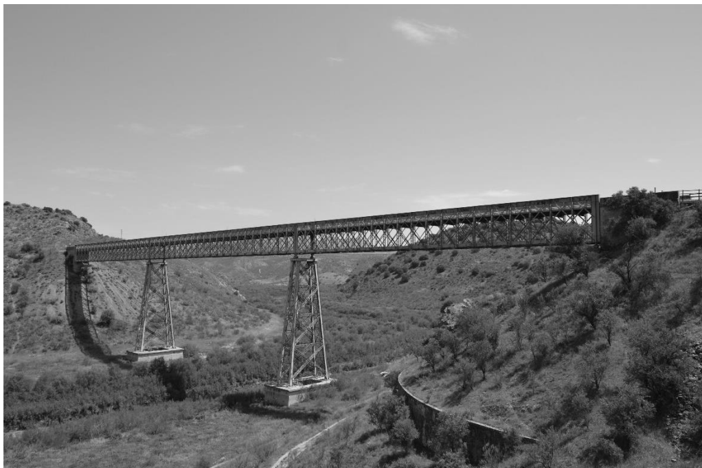
Figure 15: Guadajoz Viaduct, at the present day. Designed and built by Ch. Alessandri and A. Delaperrière, 1893. Photo: the authors.
