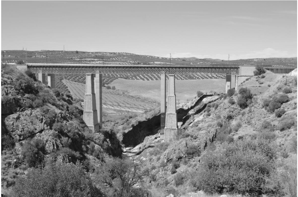
Figure 12: Río Frio Viaduct near the city of Loja, the present day. Designed and built by Jean Dupuy in 1873. Photo: the authors.
