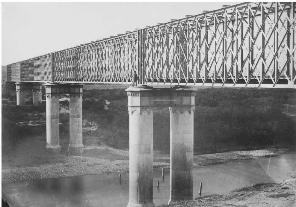
Figure 10: Guadalquivir viaduct in the Málaga-Córdoba Railway. Photo taken by José Spreafico in 1867. 55 Patrimonio Nacional, Real Biblioteca.
