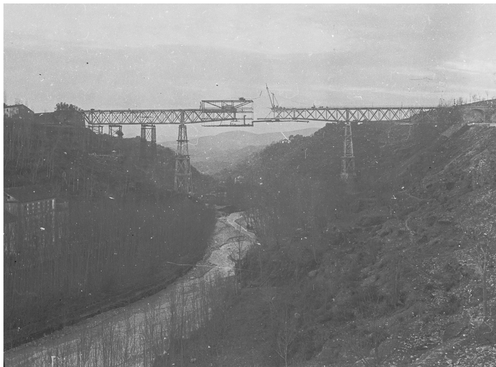
Figure 14. The second construction of the viaduct at its new site in Dúrcal (1923). Photograph taken by José Martínez Rioboo in 1925. ©Fundación Rodríguez-Acosta. Donación Martínez Sola.
