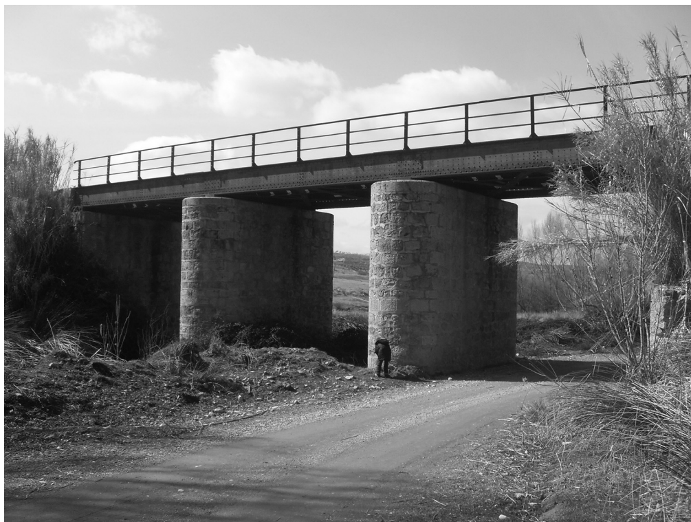
Figure 12. The definitive Gor bridge, 1909. Three 5,60 metre continuous spans. Photograph by the authors.
