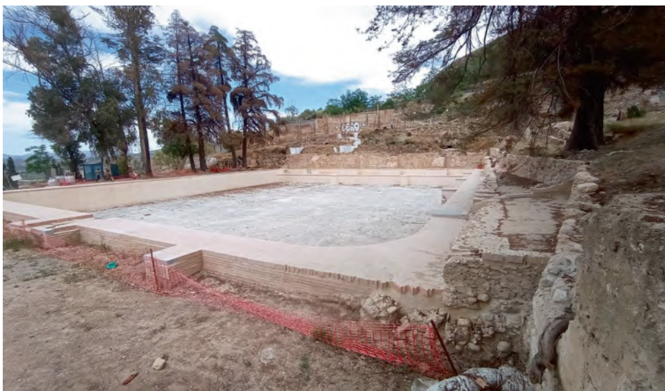
Figure 3: Photograph of the conservation work on the Nasrid pool, which was visible in Trench 1000. Figure by author García-Contreras.
