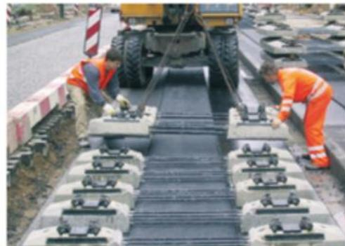
Figure 15. Placing the sleepers on the completed asphalt supporting layer [51]
