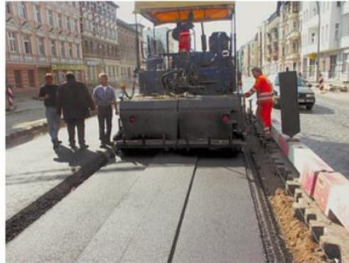
Figure 14. A paver with a special profile screed paving the top layer for the ATD-system to hold the sleepers in place later on [Source Voegelé]
