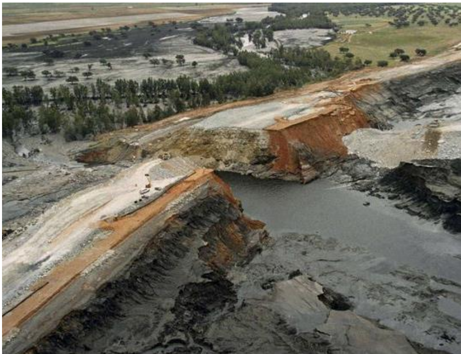
Figure 1.1. Rupture of the Aznalcóllar tailing pond dam and release of toxic tailings and acidic waters to the Agrio river. Extracted from El Confidencial 2 .
