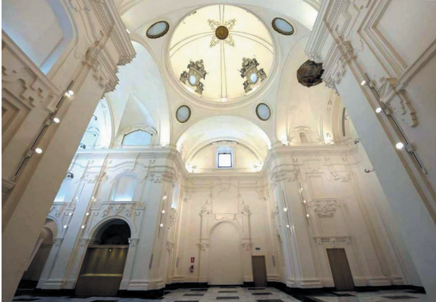
FIGURE 13.7 Francisco Hurtado Izquierdo, Oratory of Saint Philip Neri, Cordoba, 1697–1720 PHOTOGRAPHY BY JOSÉ ANTONIO DÍAZ-GÓMEZ
