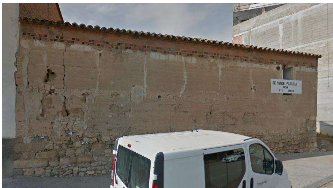
C/ Carretera No. 66
