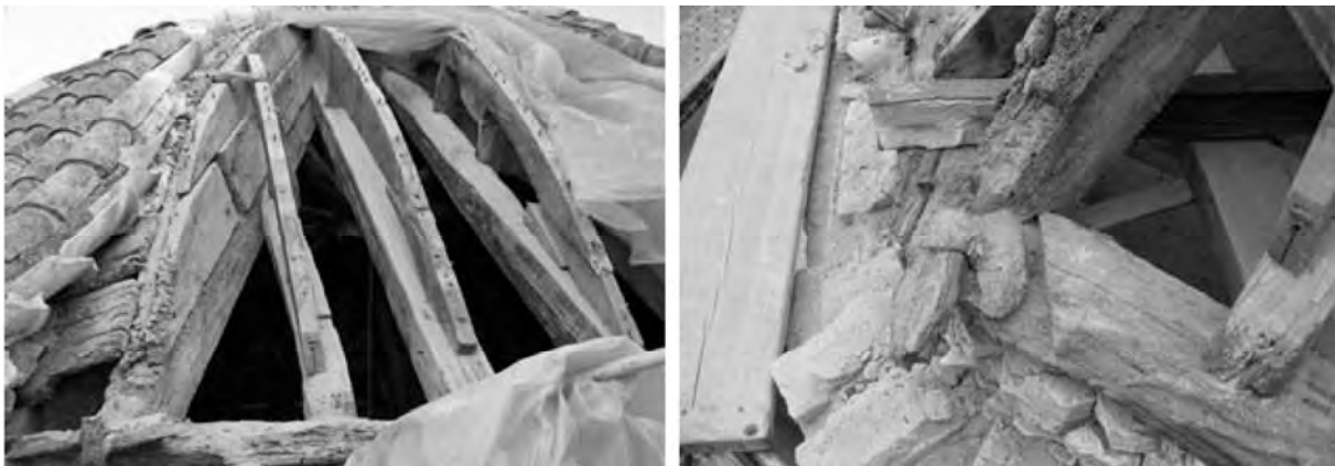
Figure 77 Original condition of the timber structure (Granero, 2009).
