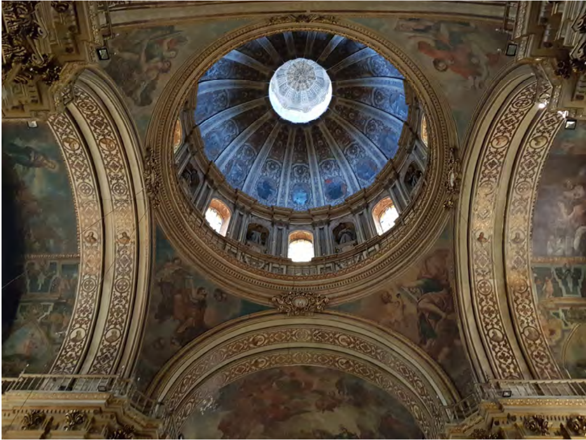
Figure 66 Inside of the church under the transept. The main arches are doubled.
