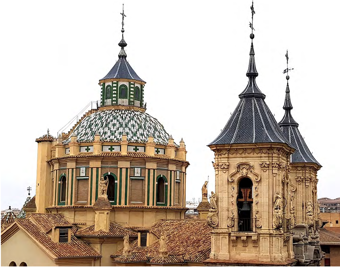
Figure 83 Dome, towers. The beautiful alboaire is seen on the cover of the dome.
