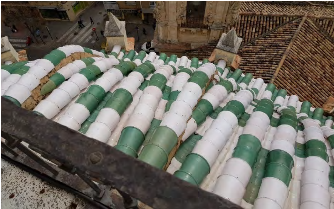
Figure 84 Tiles in the exterior of San Juan de Dios dome, with the characteristics green and white tiles of the alboaire ..
