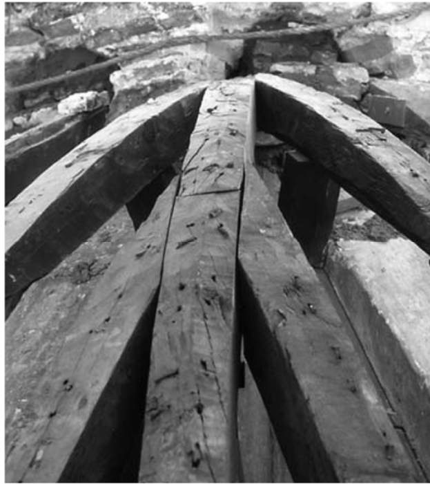
Figure 70 Union of curved rafters or camones (Pinto, 2005).
