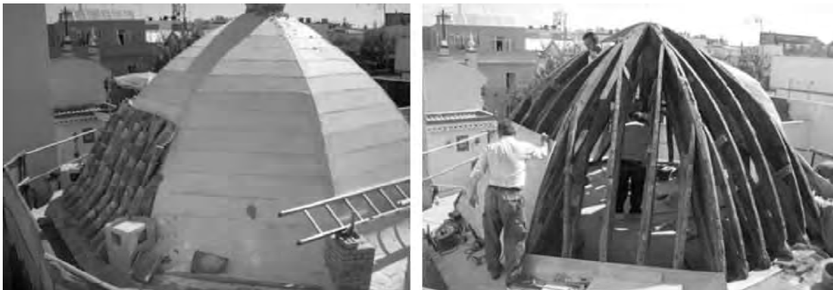
Figure 78 Structure and finishing after the restoration work (Granero, 2009).
