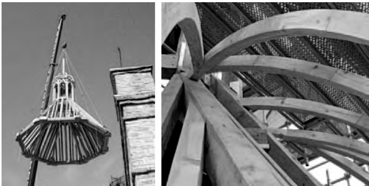
Figure 73 (left) Timber structure; (right) camones over the rafters (Vega, 2007).
