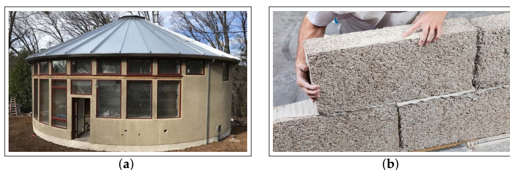
Figure 2. Hempcrete construction examples. (a) House made of hempcrete in Nevada City, CA, USA. (b) The process of building a hempcrete wall. Images taken from www.hempbuildmag.com (accessed on 15 October 2023).
