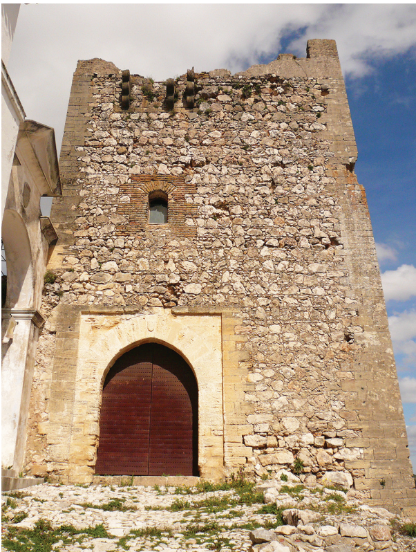
Figure 10. Tower-Gateway of the castle of Moclín.
