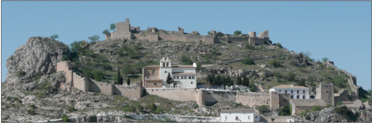
Figure 7.4 Panorama of the Castle of Moclín (Granada). On the top left, the keep, on the bottom right, the tower-gate. Photograph author's own.
