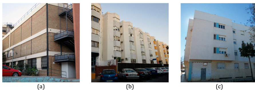
Figure 1. Façades of some of the analysed buildings: (a) C-5 (1966), (b) C-6 (1981), and (c) C-7 (2004).
