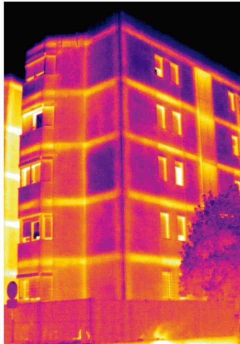
Figure 3. Thermography with thermal bridges found in the building.
