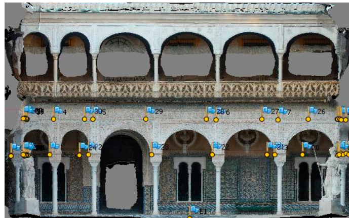
Figure 10. Control point distribution in the northeast arcade.
