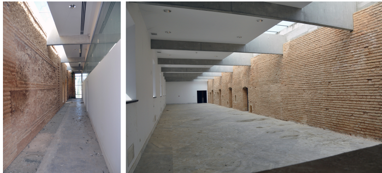
Fig. 4: Views of the civic centre annexed to the Monastery of San Jerónimo.
