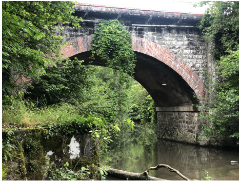
Figure 6. Examples of bridges built with different construction materials: (a) pictures from the visual inspection of a simply supported truss beam bridge; (b) photos taken during the visual inspection of masonry arch bridges.
