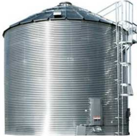
Figure 1: Typical structure of a metallic silo.
