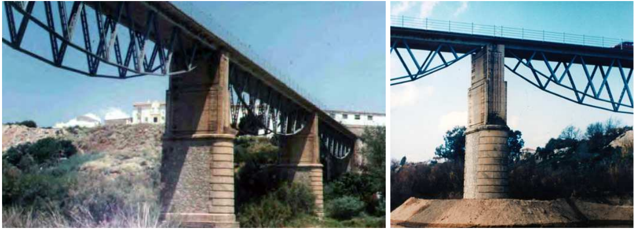
Figure 5: Photographs of the original bridge in service.
