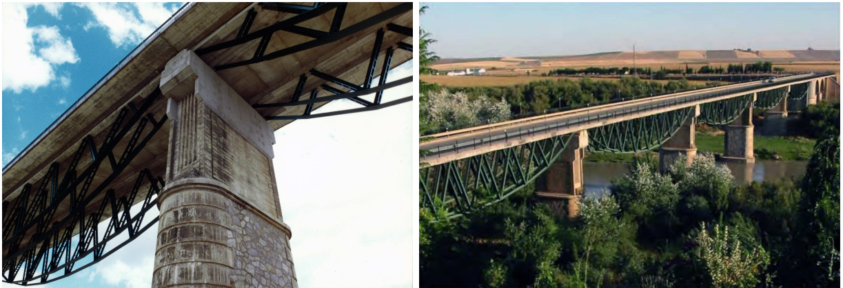
Figure 8: Views of the Current Bridge in service.
