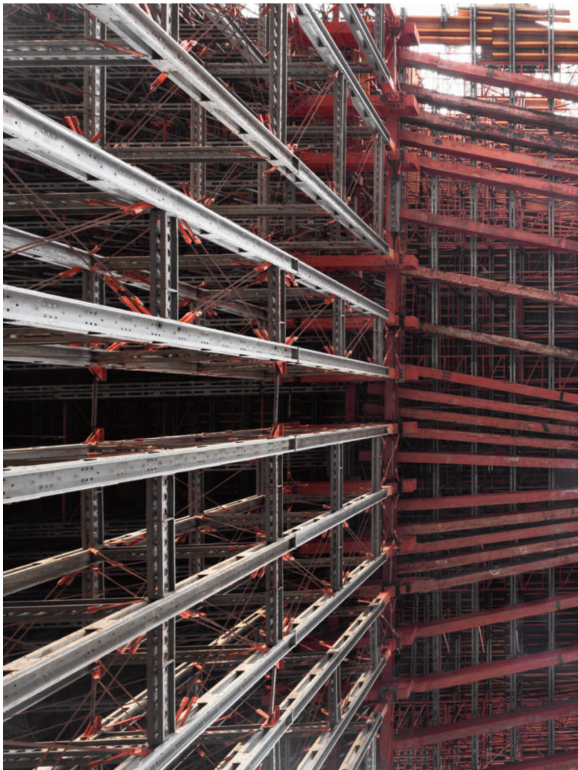
Landscape Under Construction Alfonso Batalla
