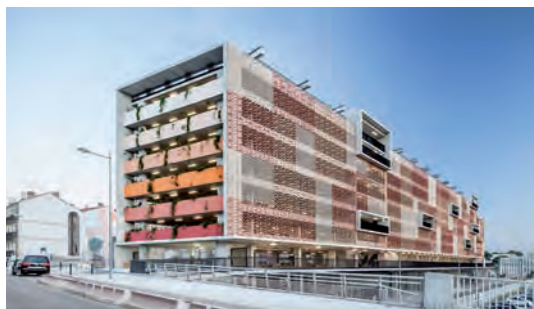
Parking Saint-Roch [LAC0121] Montpellier, Francia ARCHIKUBIK (Miquel Lacasta, carmen Santana, Marc Chalamanch)
