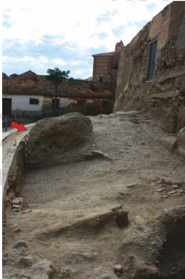
Figure 12. Remains of the bent entrance ramp with the forward bastion that protects the North Gate (Subphase Id). J. M a . Martín Civantos.
