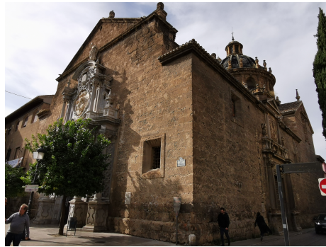
Figure 2: Main and lateral façades and dome of the church of San Justo y Pastor.
