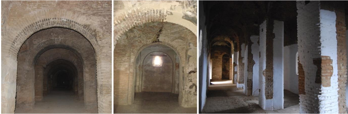
Figure 8. Brick pilasters of the defensive towers
