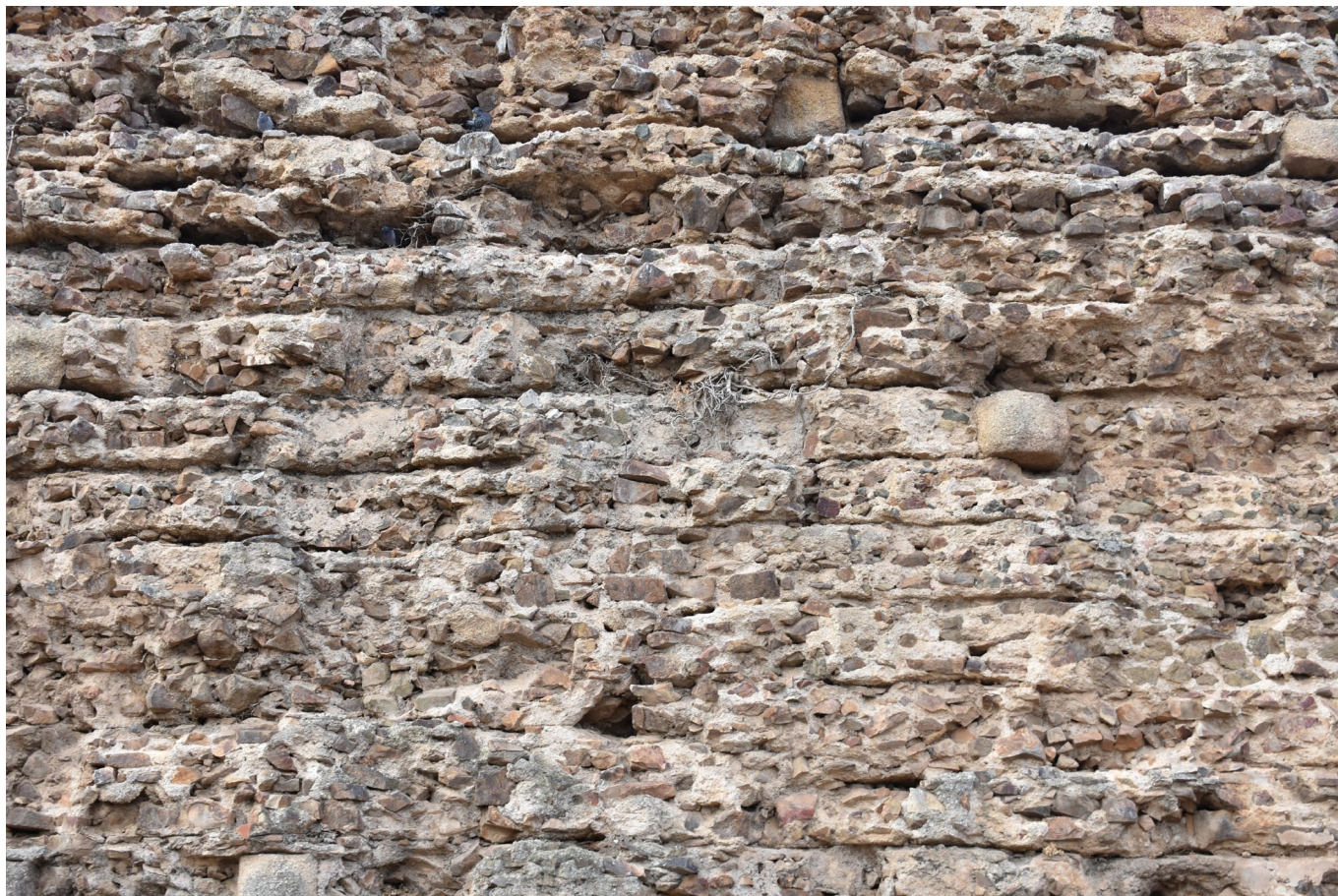
Figure 1. Superimposed layers of mortared rubble as the structural core ( opus caementicium ) of the theatre of Augusta Emerita (Mérida, Spain). Image by the author.
