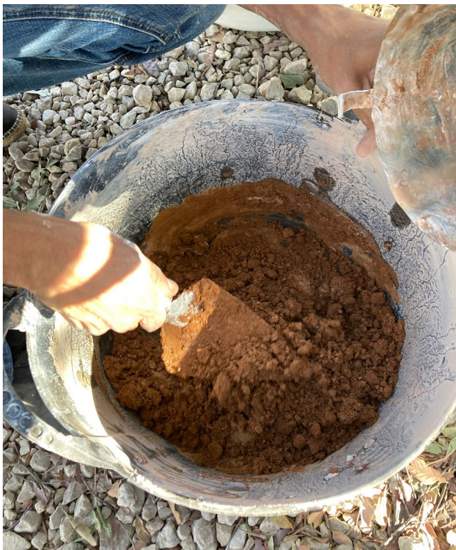
Figure 3. Water added to a mortar mix. Photo taken during the 2021 opus signinum recreations of the AQUAROLE project, at the Lime Museum of Morón (Seville). Image by the author.
