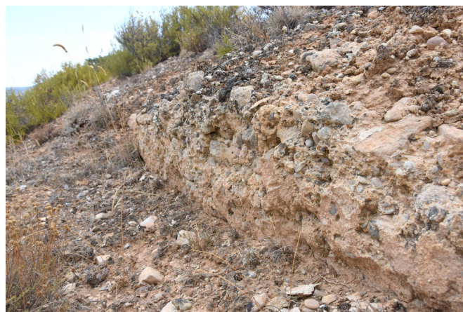
Figure 7. Detail of the limewash preserved on the walls of the aqueduct at the site of La Paeriza. Image by the author.
