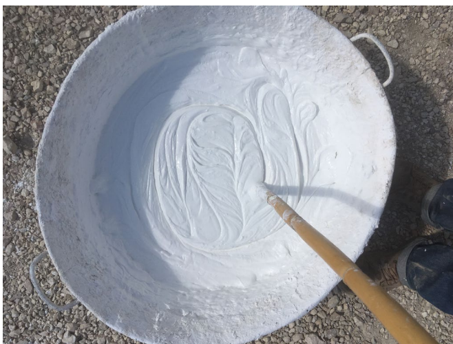
Figure 4. Lime slaking: lime putty after the addition of water to nuggets of calcined limestone (quicklime). Photo taken during the 2021 opus signinum recreations of the AQUAROLE project, at the Lime Museum of Morón (Seville). Image by the author.
