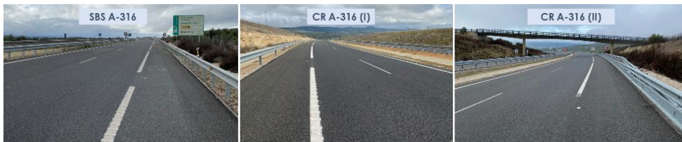
Figure 4.2.3. Aspects of the surface asphalt layers manufactured with SBS and crumb-rubber-modified binders on A-316 highway after 63 months of service life.
