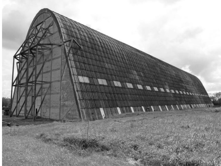
Figure 1.24. Ecausseville airship hangar. Exterior
