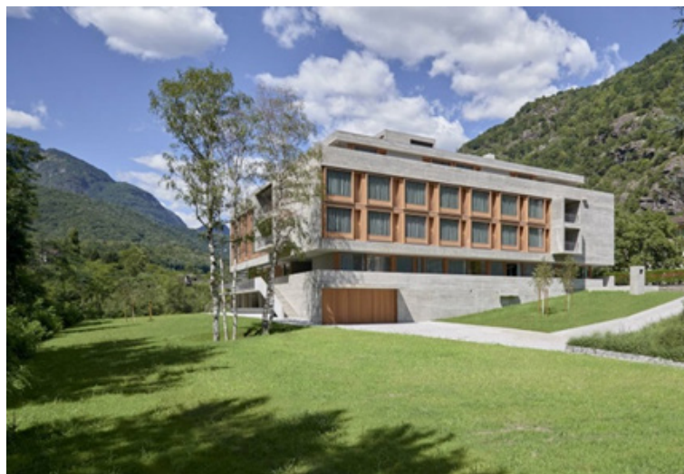
Figure 1.53. the “Elena Cerio” Retirement home, Giornico, Switzerland (photo by Pedrazzini Guidotti sagl, Lugano)
