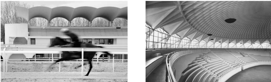
Figure 1.6. Zarzuela Hippodrome, E. Torroja, 1941 (left) and Sports hall in Rome, P. L. Nervi, 1957 (right)
