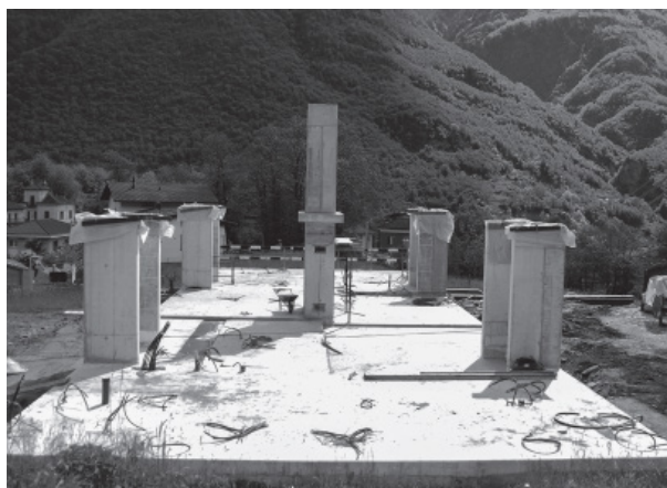
Figure 2.57. Supporting RC elements (Photo by Tocchetti and Pessina)
