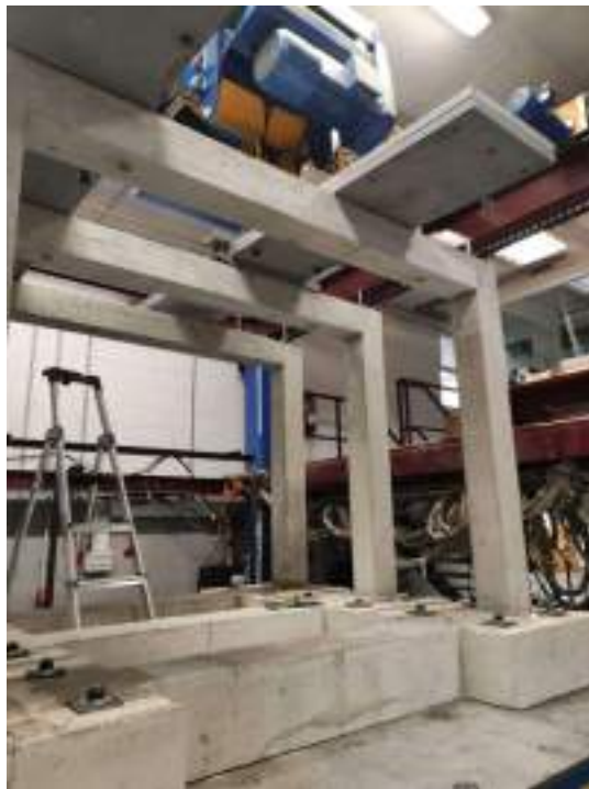
(a) Frontal view of the reinforced concrete frames, before the construction of the walls.
