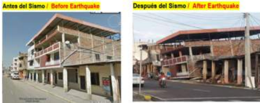
Figure 1.3: Example of a structural collapse due to the MIF irregular vertical distribution of stiffness (Landívar, 2016).
